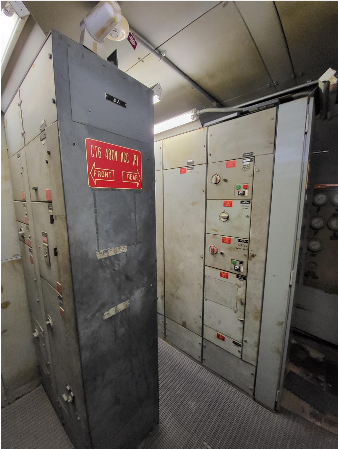
Current CT6 cab – northern half (showing LV MCCs)
